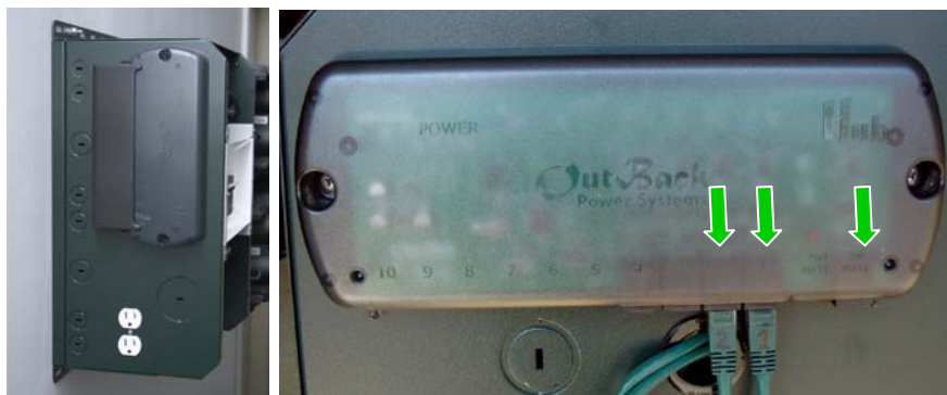
Figure 20 Mounted HUB with cover (left) & HUB connected to 2 inverters (right). The far right arrow shows where the MATE connects.
