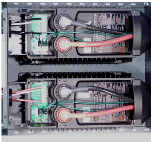
Figure 15 Inverter wiring without DCC.
